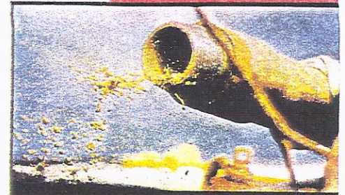
Blowing dirt and debris from the pipe.
